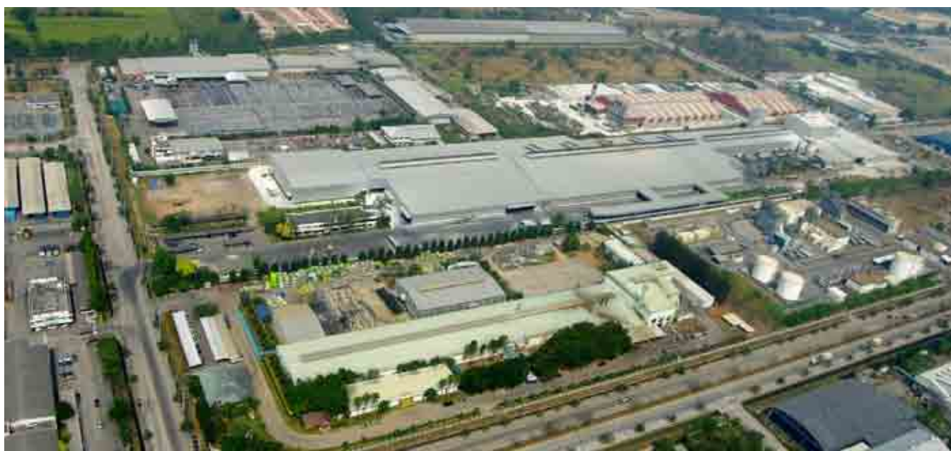
Scene of regional development: Saraburi Industrial Zone
